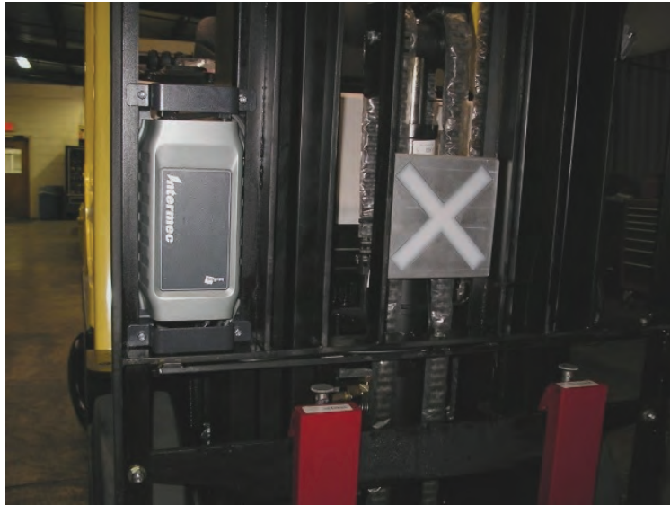
IV7 and Antenna Mounted on ALBR: IV7 is placed in end channel, with antenna in center for best tag reading in this installation.
