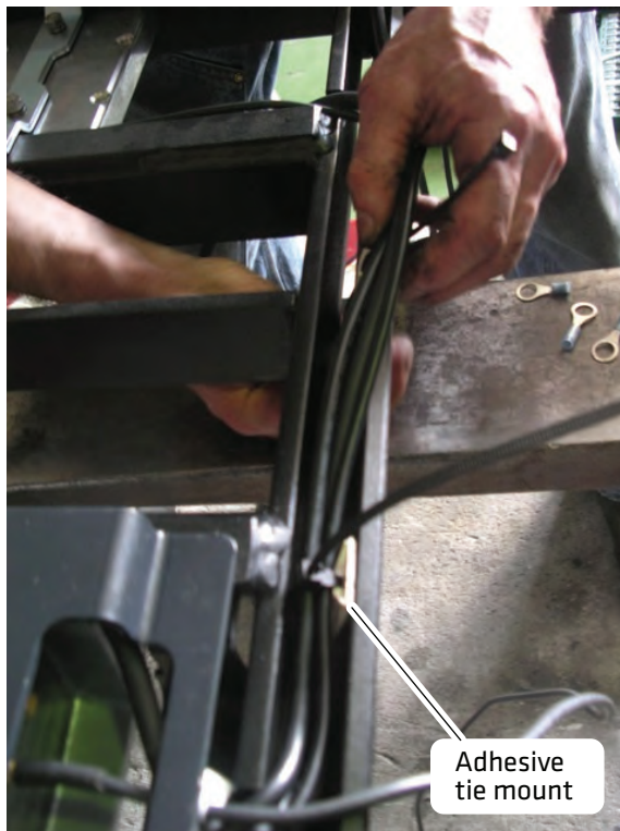
Installing Cables in ALBR Cable Tray
